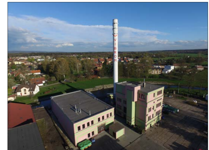
Fig. 1 Vibrom's production facility in the Czech Republic
